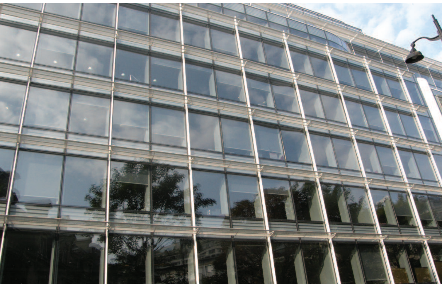
Unibail-Rodamco, the largest real estate company in Europe, added internal blinds made of Dickson Sunworker fabrics for its Paris headquarters as part of an energy management program.
